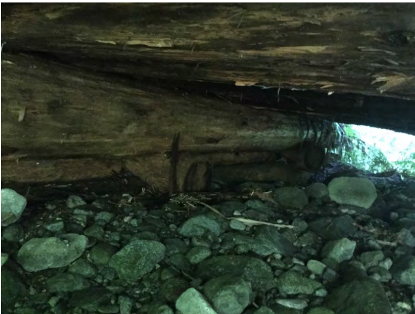
Left Bank Abutment
