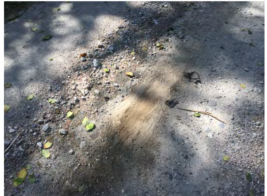
Stringer Protruding Through Deck at Left Abutment
