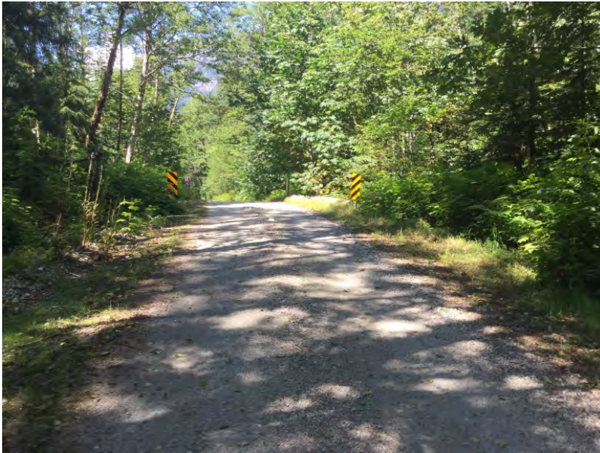
Left Approach Facing Bridge
