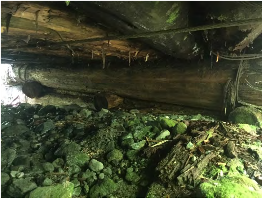
Right Bank Abutment
