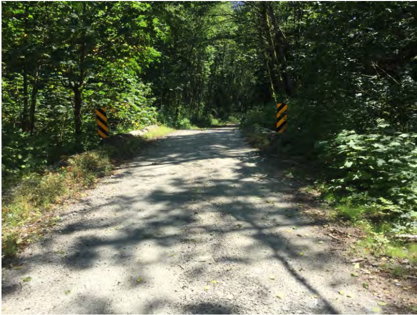
Right Approach Facing Bridge
